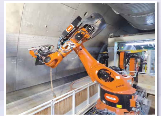
▲ 管理局團隊於茶果嶺隧道內參觀全自動的敲鑿及鑽孔機械臂，布依格的機械工程師為管理局團員介紹操作員如何遙距控制機械臂於隧道內的工作，將噪音及塵埃的危害徹底消除。 Inside the Cha Kwo Ling Tunnel, the Board's delegation visited the fully automated robotic arm for concrete scrubbing and drilling. The Plant Engineer of Bouygues explained to delegates how the operator could remotely control the work of the robotic arm inside the Tunnel to completely eliminate the noise and dust hazards.
