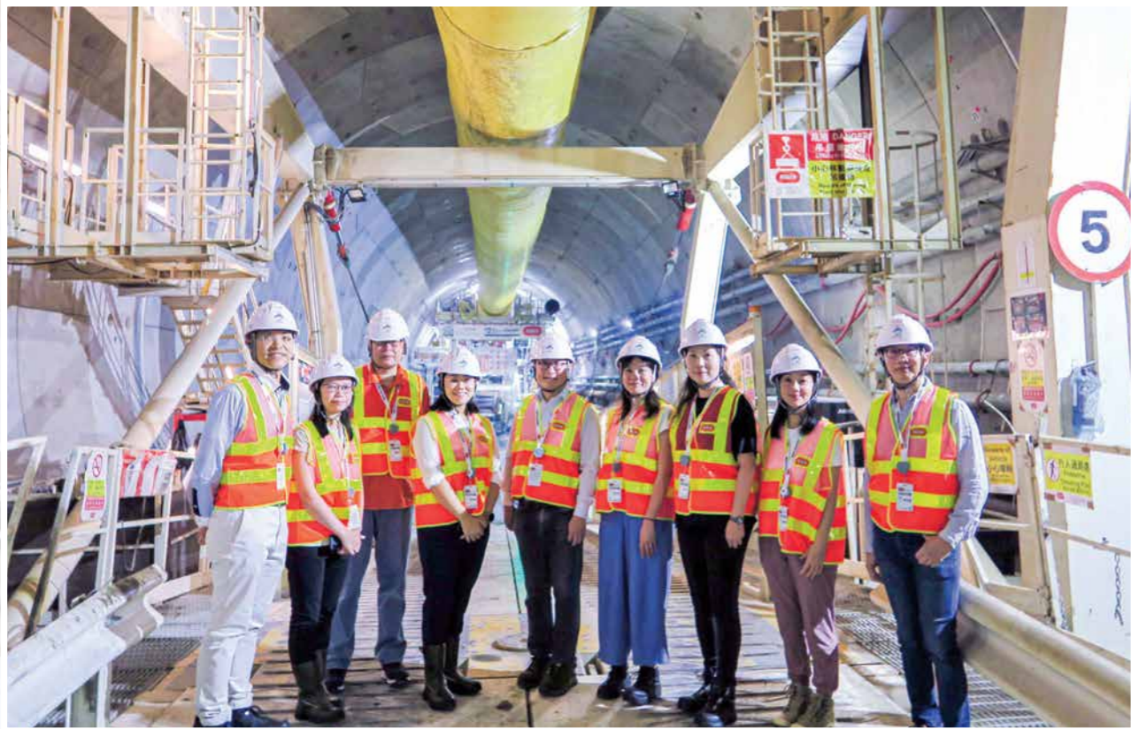
▲ 管理局團隊攝於建築中的茶果嶺隧道內，探訪團員包括：主席曾浩輝醫生，銅紫荊星章(中)、醫管局代表高嘯軒醫生(左一)、勞工處勞工事務主任岑淑怡女士(左二)、僱員代表周思傑先生，榮譽勳章(左三)、僱主代表張瑞祺女士(左四)、管理局時任營運監督陳英偉先生(右一)、管理局聽力學家黎珮珊女士(右二)、管理局行政總監吳惠英女士(右三)及僱主代表黃詩岸女士(右四)。 The Board delegation photographed inside the Cha Kwo Ling Tunnel under construction, with visiting delegates included: ODCB Chairman Dr Thomas Tsang, BBS (Centre), Hospital Authority representative Dr Ko Siu-hin (1 st from left), Labour Officer of Labour Department Ms Joey Sham (2 nd from left), Employee Representative Mr Chau Sze-kit, MH (3 rd from left), Employer Representative Ms Debbie Cheung (4 th from left), former ODCB Director of Operations Mr Alfred Chan (1 st from right), ODCB Audiologist Ms Sandy Lai (2 nd from right), ODCB Executive Director Ms Erica Ng (3 rd from right), and Employer Representative Ms Caroline Wong (4 th from right).
